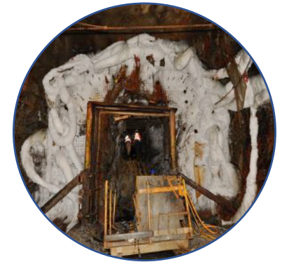
If Necessary Freezing Any Unstable Ground Above Crosscut
