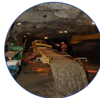
Crosscut Material Processed by Water Wash Plant Underground
