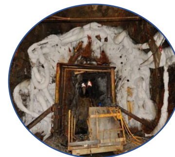
If Necessary, Freezing Any Unstable Ground Above Crosscut
