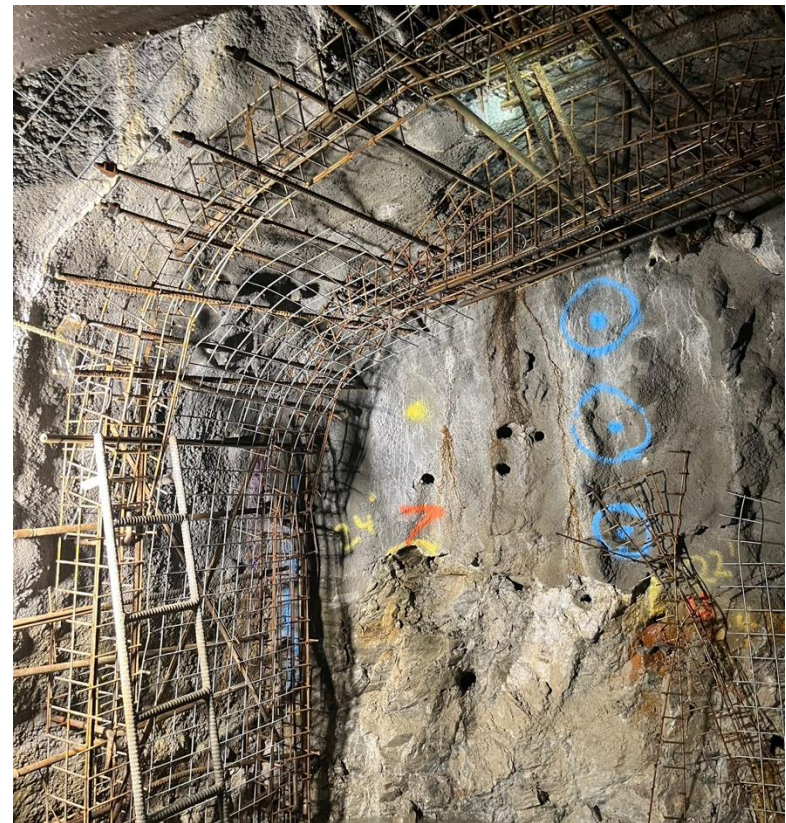
Shotcrete Arch Support
