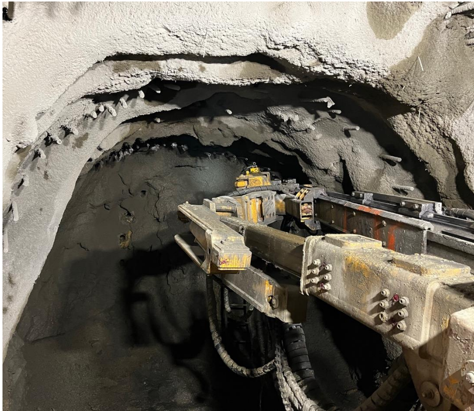
Shotcrete and Spilings at Crosscut Heading
