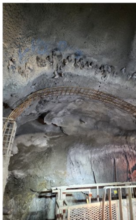
Shotcrete Arch Form, Spilings Drilled Above
